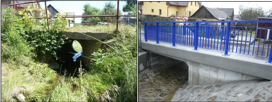
Figure 1 Kozlov bridge before reconstruction and after reconstruction
