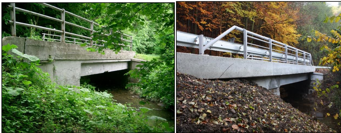
Figure 2 Stupava bridge before reconstruction and after reconstruction
